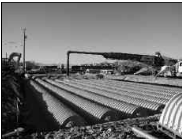
Placing stone with the conveyor boom extended.
