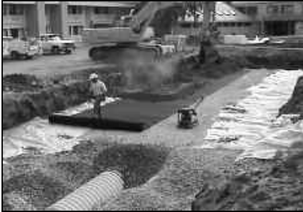
Roll out filter fabric over the angular stone.
