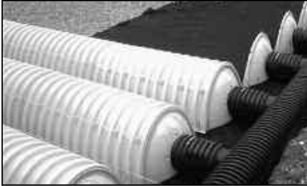
Scour protection fabric at manifold.
