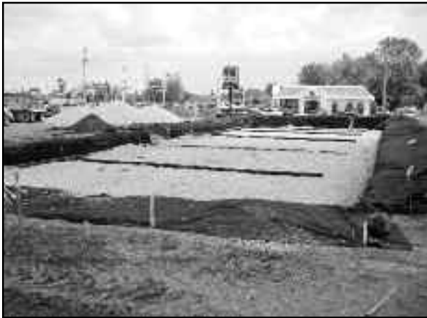
Filter fabric and underdrains installed.
