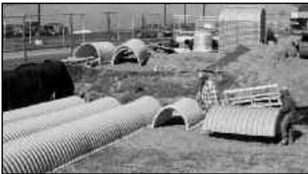
Maintain a minimum of 6" (152 mm) between chamber feet.
