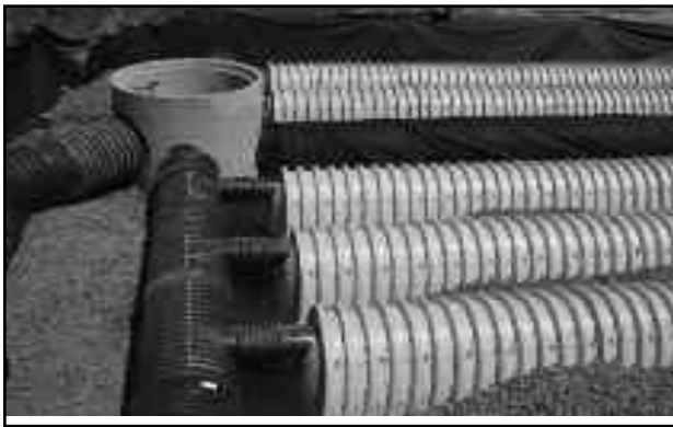
Scour protection fabric at manifold.
